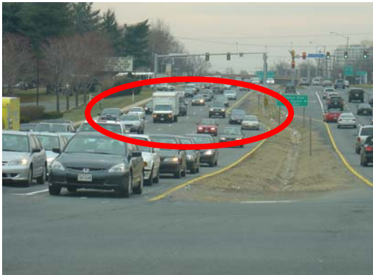
Figure 7. Low Volume Critical Movements (in this case, main line left turn vehicles, as circled, are spilling over into the adjacent through lanes)
