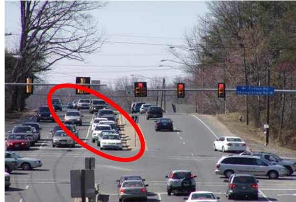
Figure 7. Low Volume Critical Movements (in this case, main line left turn vehicles, as circled, are spilling over into the adjacent through lanes)
